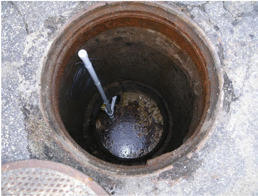
Outlet Manhole Installation
