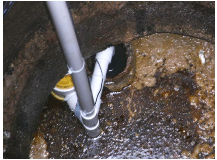
Flood Sensor Placed in tee to Detect High Water
