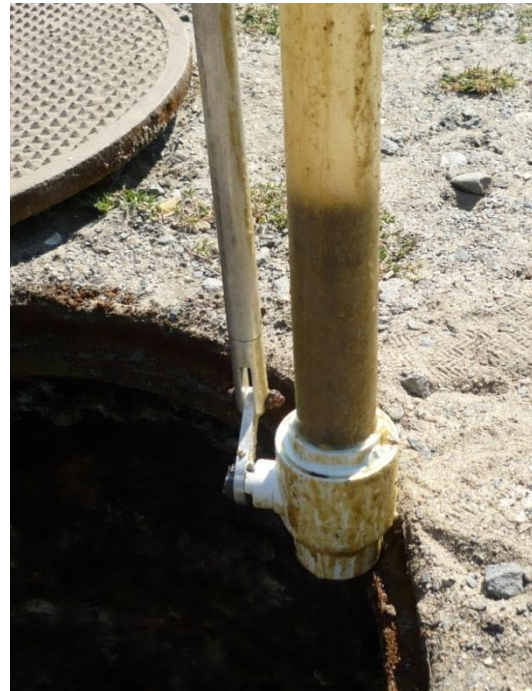
Solids Settle on Tank Bottom
